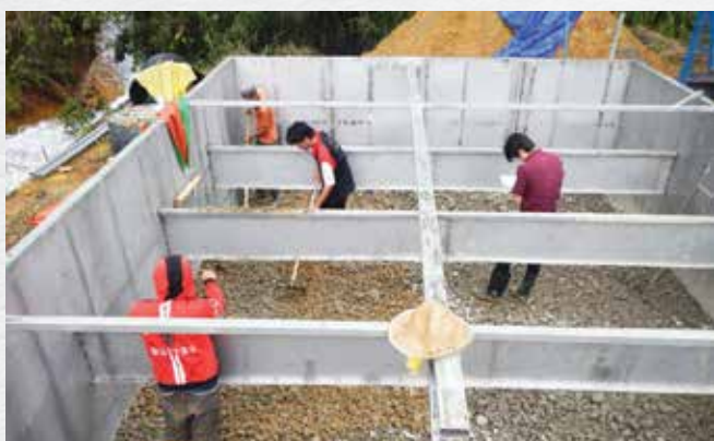
Penyediaan loji pandu rawatan pasif AMD Preparation of AMD passive treatment pilot plant
